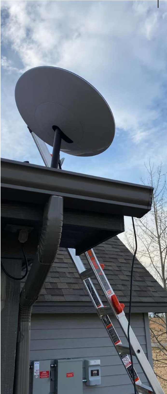
On the roof (50km protection)
